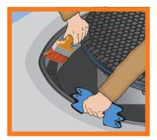
The frame seating face should be brushed and cleaned every time the cover is lifted.
